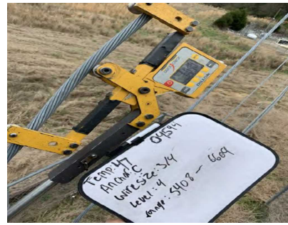
Anchor C Guy Level 3R
